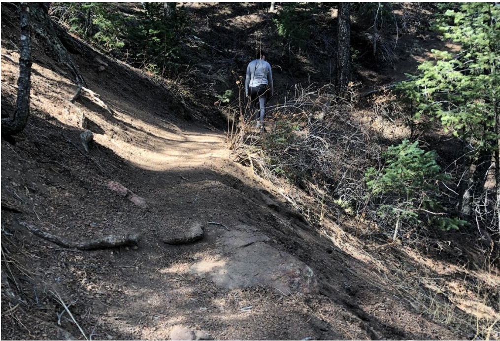
Segment E2 – Trail Maintenance section on Hiking Only Trail
