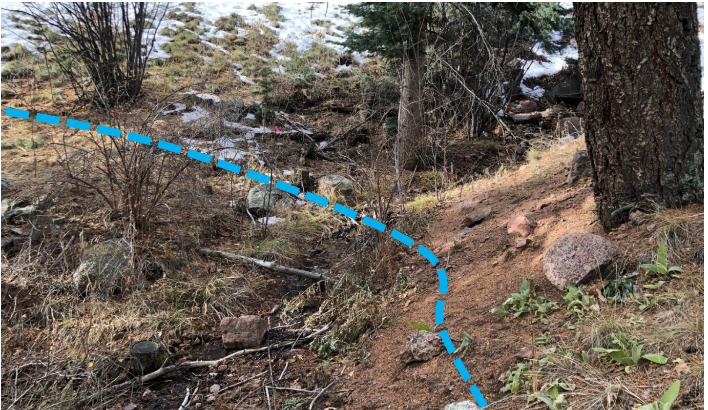
AN10 creek crossing with new culvert
