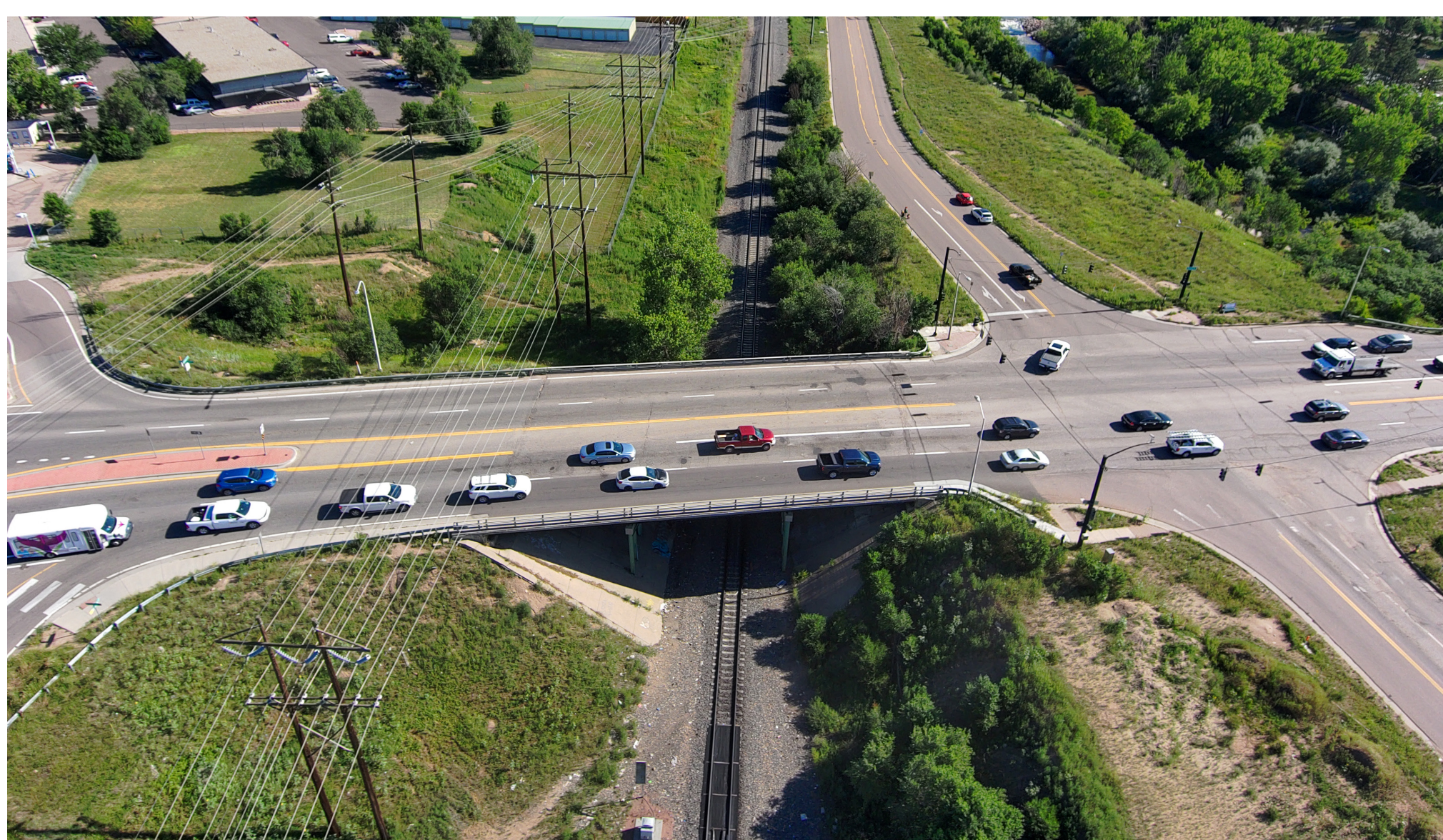
Railroad Bridge looking north.
