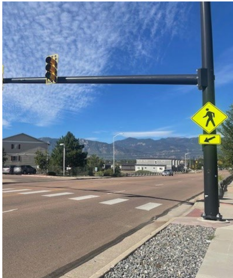
Celton Rd. new crosswalk and pedestrian signalization
