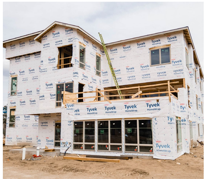
Affordable housing construction at South Murray Boulevard
