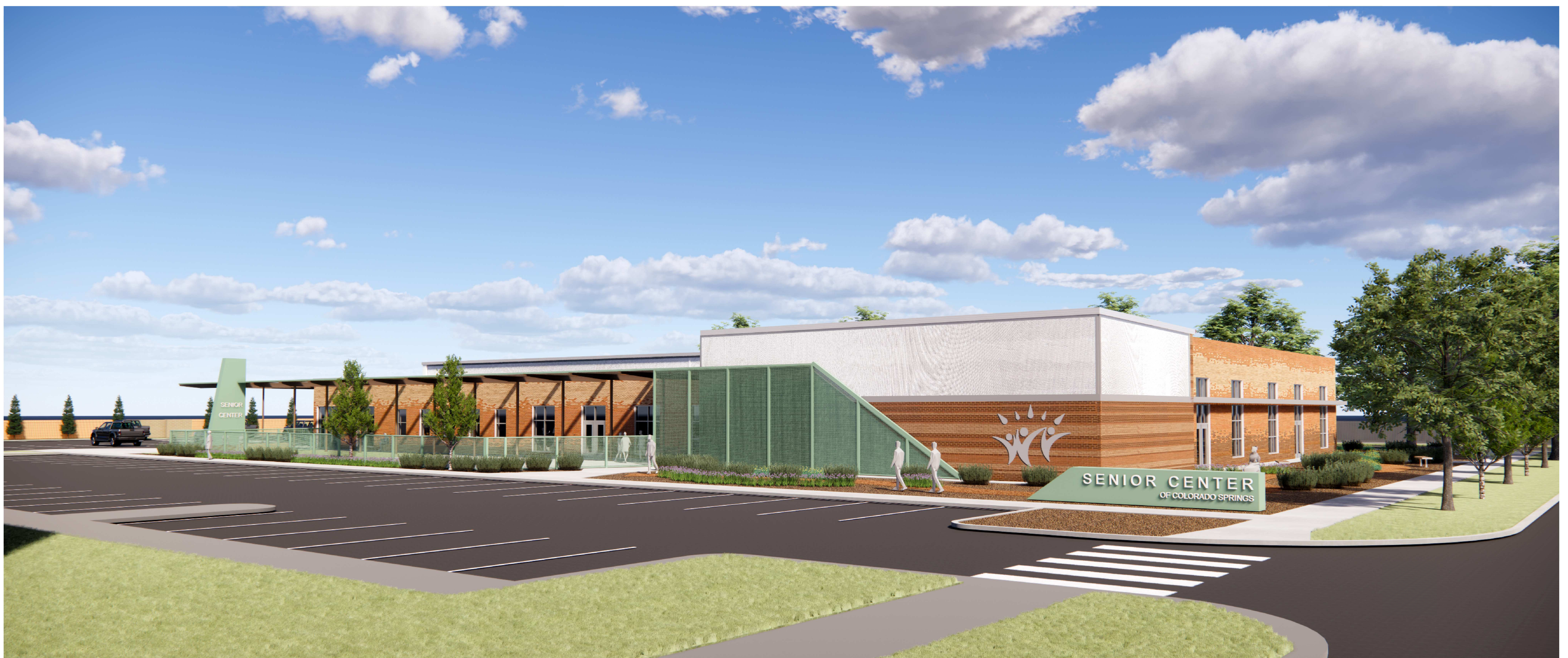
VIEW FROM HANCOCK AVE.
